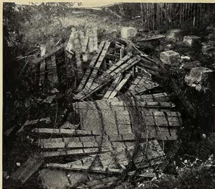
FIG. 8. Demolished tank west of the south end of Honaunau School, footings on which the tank formerly stood, and part of the school building, from the southwest.
